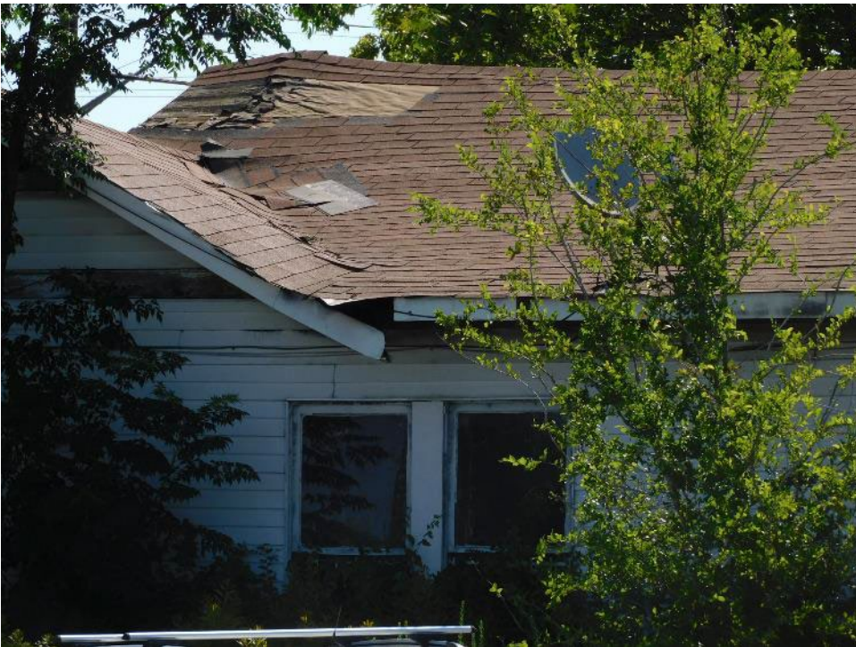
Photo 12, Exterior, damaged roof, east elevation.
